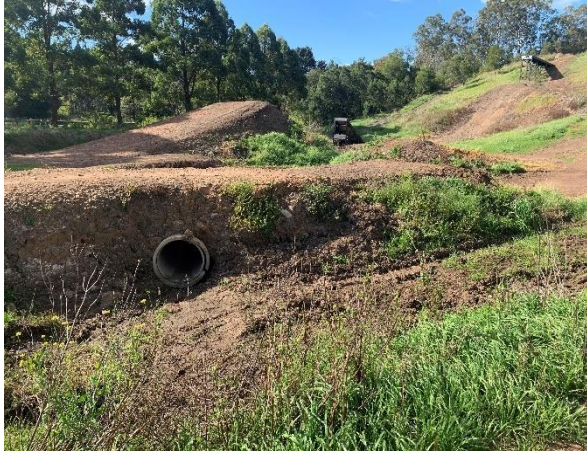
Figure 10: Drainage pipes incorporated into access tracks
